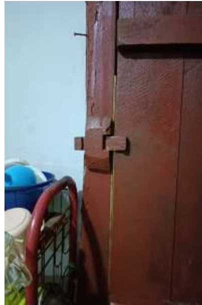
Picture 17 Doors and locks knock down Loa Tjong Sin House
