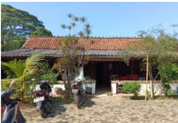
Picture 13 Front View of Kebaya House of Loa Tjong Sun
